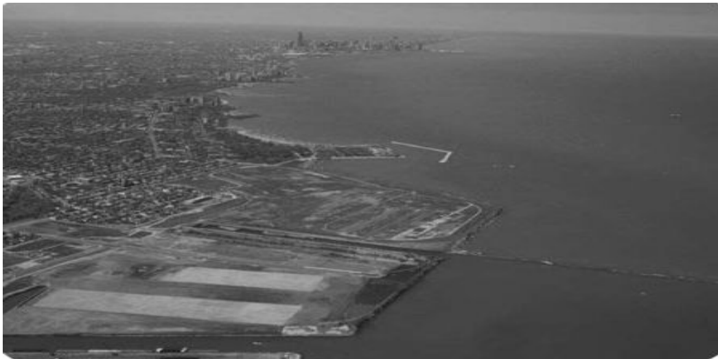
An aerial view of the northern half the site after most the mill was demolished in 1995. Large plots of vacant land dominate the landscape only 12 miles from downtown. (Photo by Okrent Associates, provided by Pamela Austin, McCaffery Interests)
